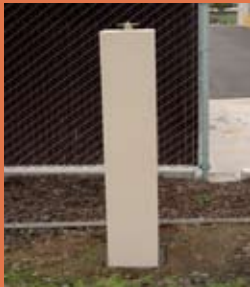
Place Decorative Column over lower post section, Slide upper section into post and secure with attachment rod.
